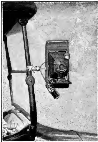
The Optipod holds the camera; the Tin.er trips the shutter
